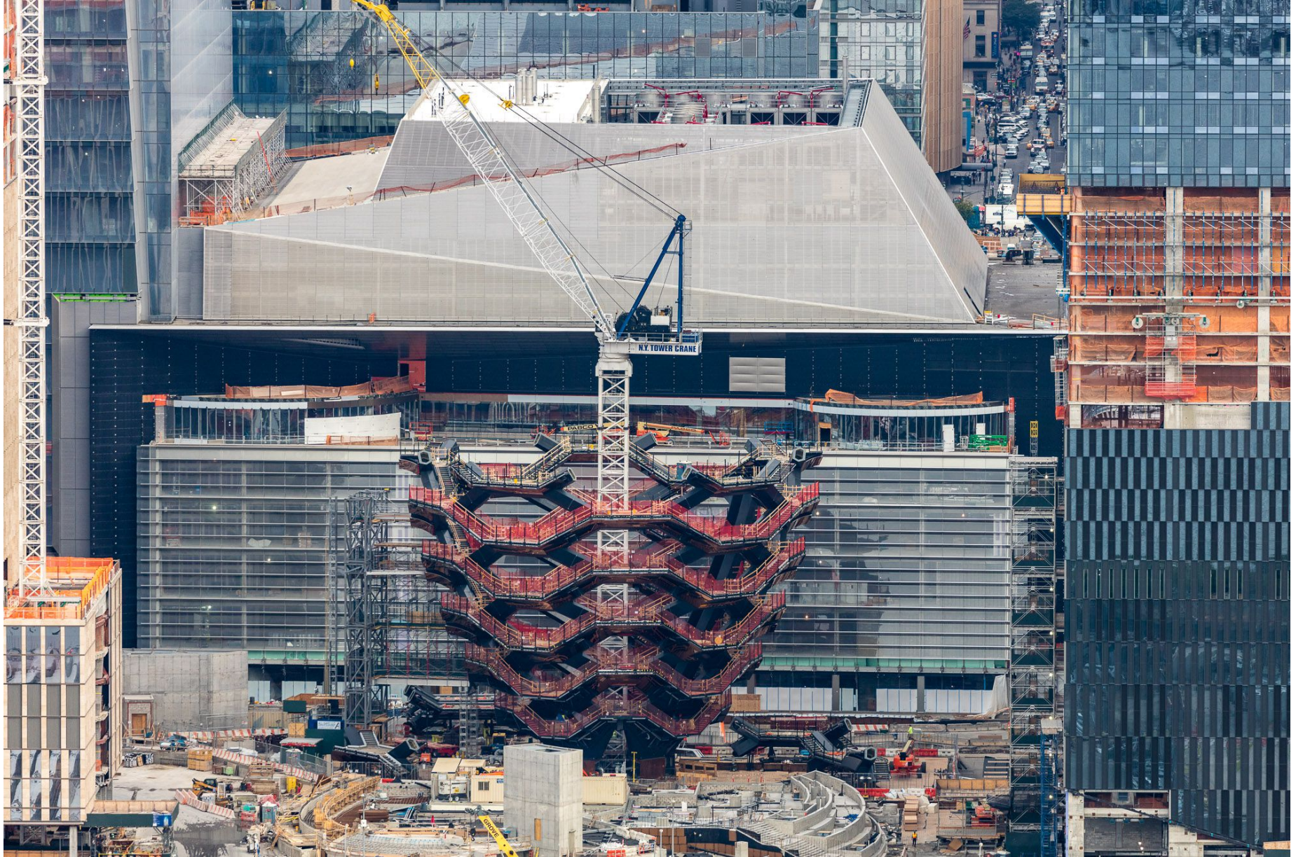
Thomas Heatherwick's Vessel on the rise in Hudson Yards.
