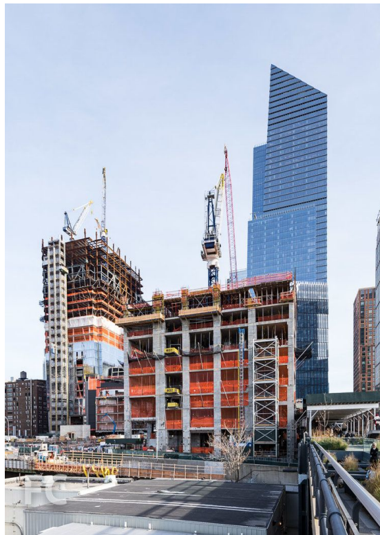
15 Hudson Yards and the Shed under construction Field Condition
