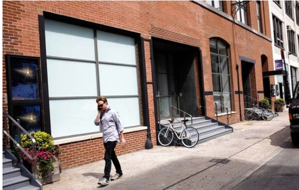
The space at 525 W. 25th St. for Driscoll Babcock Galleries.
